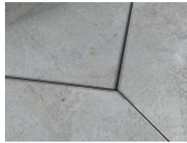
Y Joint Detail New type
