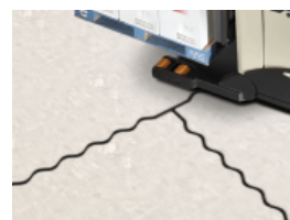
Sinusoidal T Joint Detail
